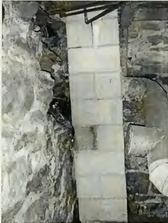
Figure 12 New Chimney and Disturbed Stonework in southeast corner of Basement, 2002
